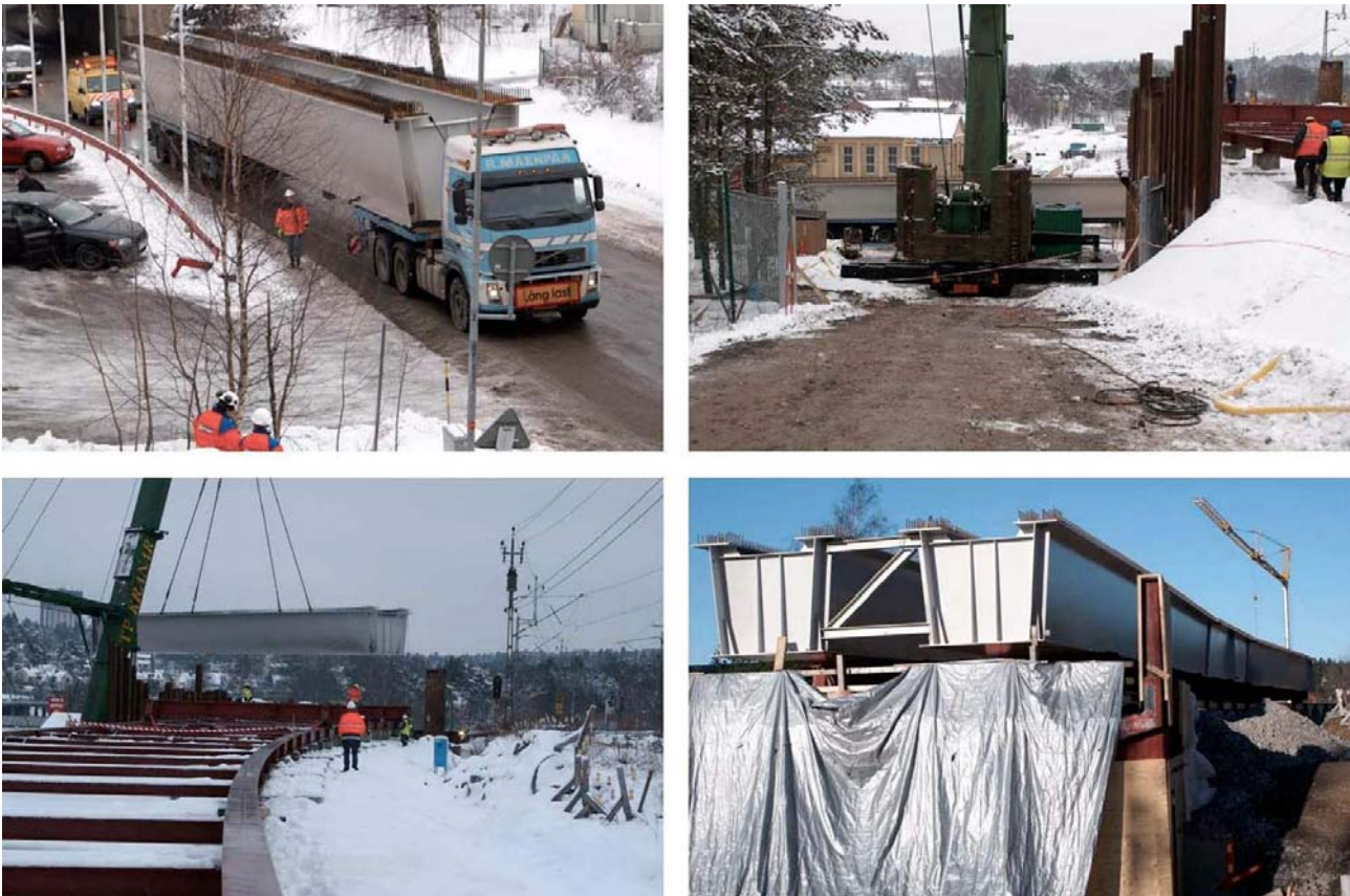
Figure 7. The arrival of the steel girders from Finland and the lifting operation from truck to launching track behind the abutment structure.
