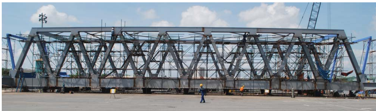
Figure 12. Assembly of the lifting bridge section in a deep water port.
