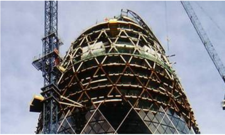
Figure 8. Facade construction of the 30 St. Mary Axe (Courtesy of J. Fernandez).
