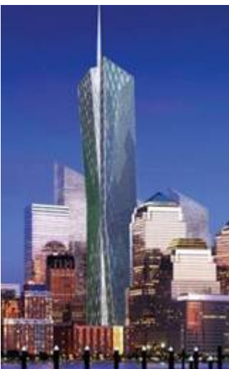
Figure 9. Facade construction of a diagrid tall building (Courtesy of L. Szewczyk and I. Lee).
